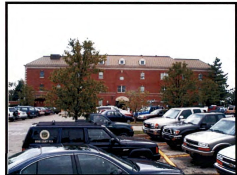
Plate D: View of 1980 Boone County Administration Building from proposed new site
