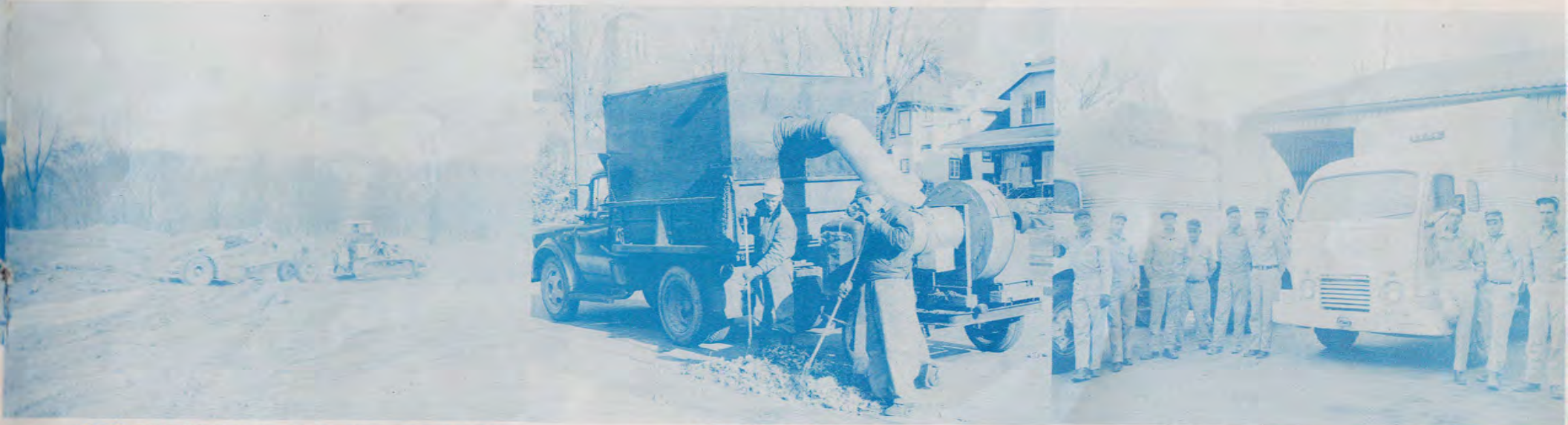
NEW LEAF VACUUM Built by City as an attachment to brush chipper.
