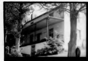
Two room log section and stone foundation under porch
