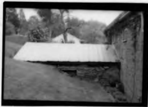
Stone cellar (rear)
