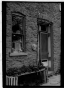
Fenestration and detail
