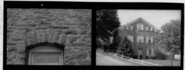
North elevation and masonry detail
