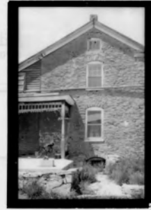
detail, southeast elevation
