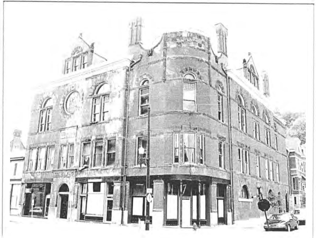
Photo 2 (Left) The Cox Building, MSM-III Mason County, Ky. North (3rd St) Facade, Looking SSE Orloff Miller, 2007, author's collection
