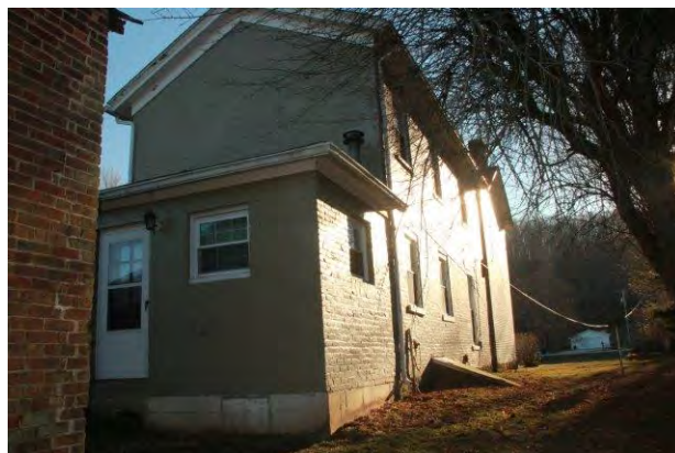
One-story 1970s addition
