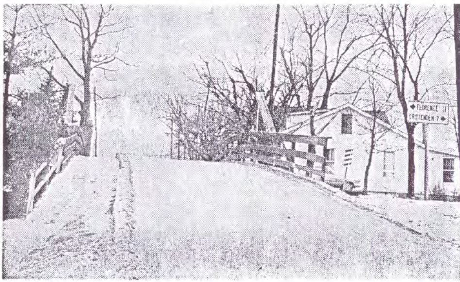
ANCIENT BRIDGE on Kentucky 16, that goes from Walton to Verona, is barely wide enough for two cars. It crosses the L. & N. tracks.
