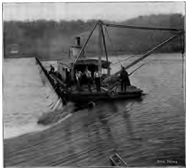
FIG. 6. DERRICK BOAT OPERATING MOVABLE DAM NO. 4.
