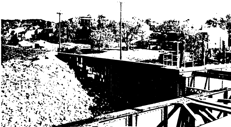
Part of Earth, Steel, and Concrete Construction used under Bridge and roadways. Here L & N Railroad area.
