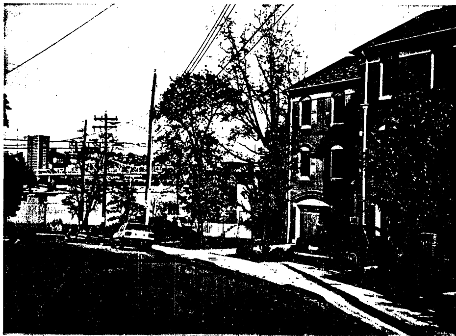
Shelby Street along Licking River not flood protected. Units sell for $265,000.
