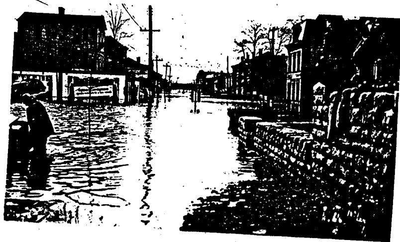
Water stops at 3rd. & Washington Srtreet Picture looking west from Mansion Hill
