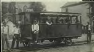
This is how the passenger traffic was handled on the Carrollton some 27 years ago. The man at the controls right is George W. King, present day engineer for the little road.
