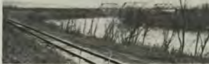
Above: The Carrollton's section gang under former Foreman Taylor Browning laid a job of new track to serve the nearby principal industry—the Nuygen Sand Company. Left: The construction of the Carrollton and the Old Reliable at Worthville, Ky. The Carrollton's track is on the left; the L. & N.'s bridge across the Kentucky River may be seen in the distance.
