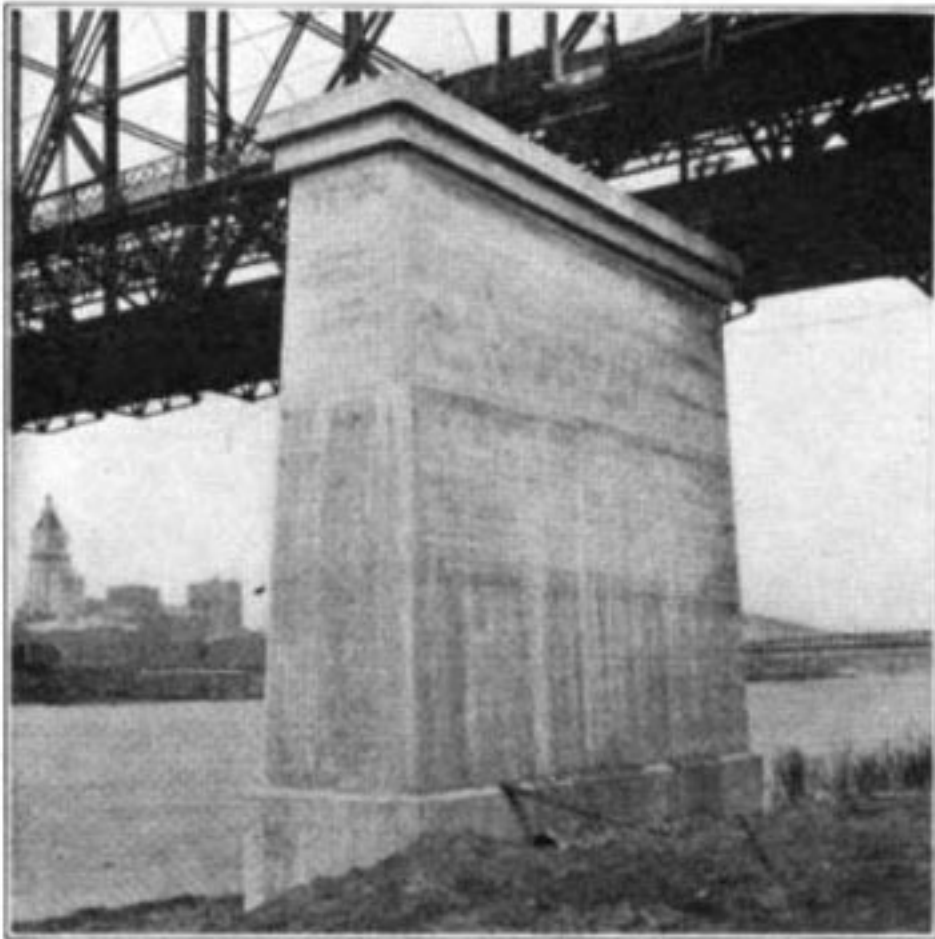
The Completed South Shore Pier for the River Bridge
