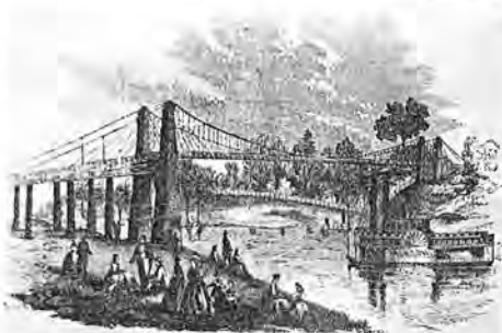
Suspension Bridge over the Licking River.
