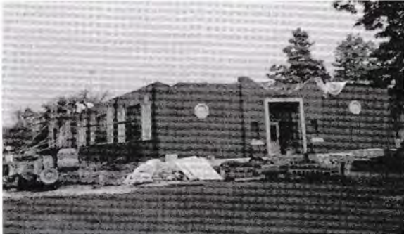
Addition of School 2nd Floor
