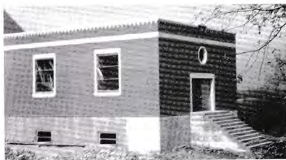
Construction of "Children's Chapel"
