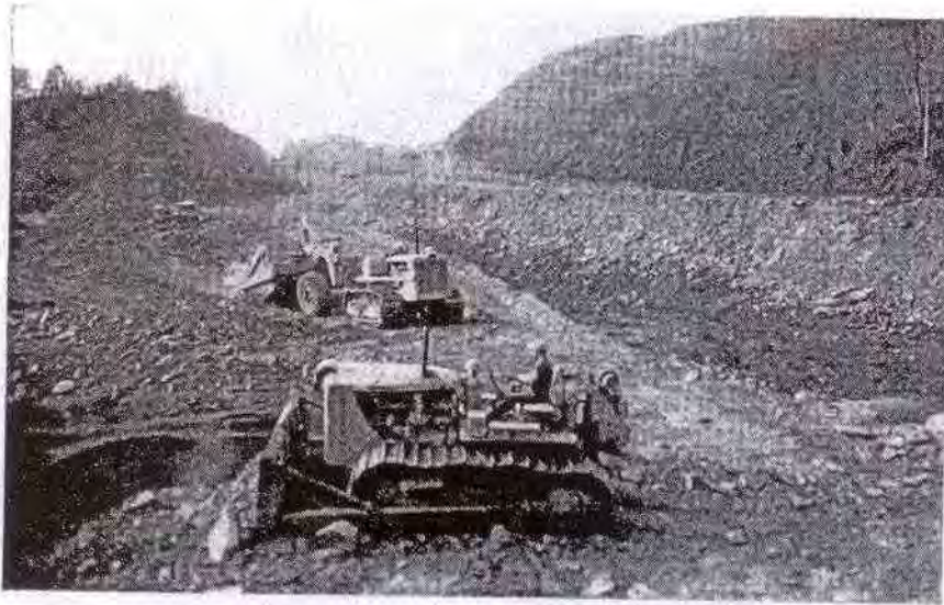
Left: Earth-moving machines have here made a good start in grading for relocating line. Former trackage was to the left, just out of camera range. Below, left: Workmen have assembled big, multi-plate pipe and it is now ready to receive over-burden of earth and rock. Below, right: With pipe in place and work of relocating line completed, a freight train passes over new track.
