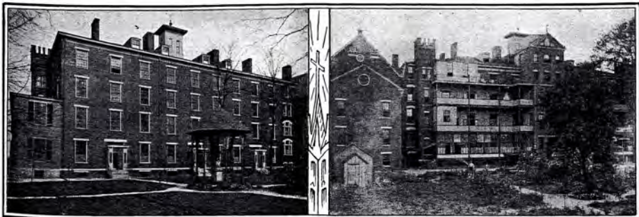
(Left) Old Baptist Theological Seminary (side view). (Right) Hospital of the Sisters of the Poor of St. Francis (side view), on Eleventh Street, Covington, Ky.
