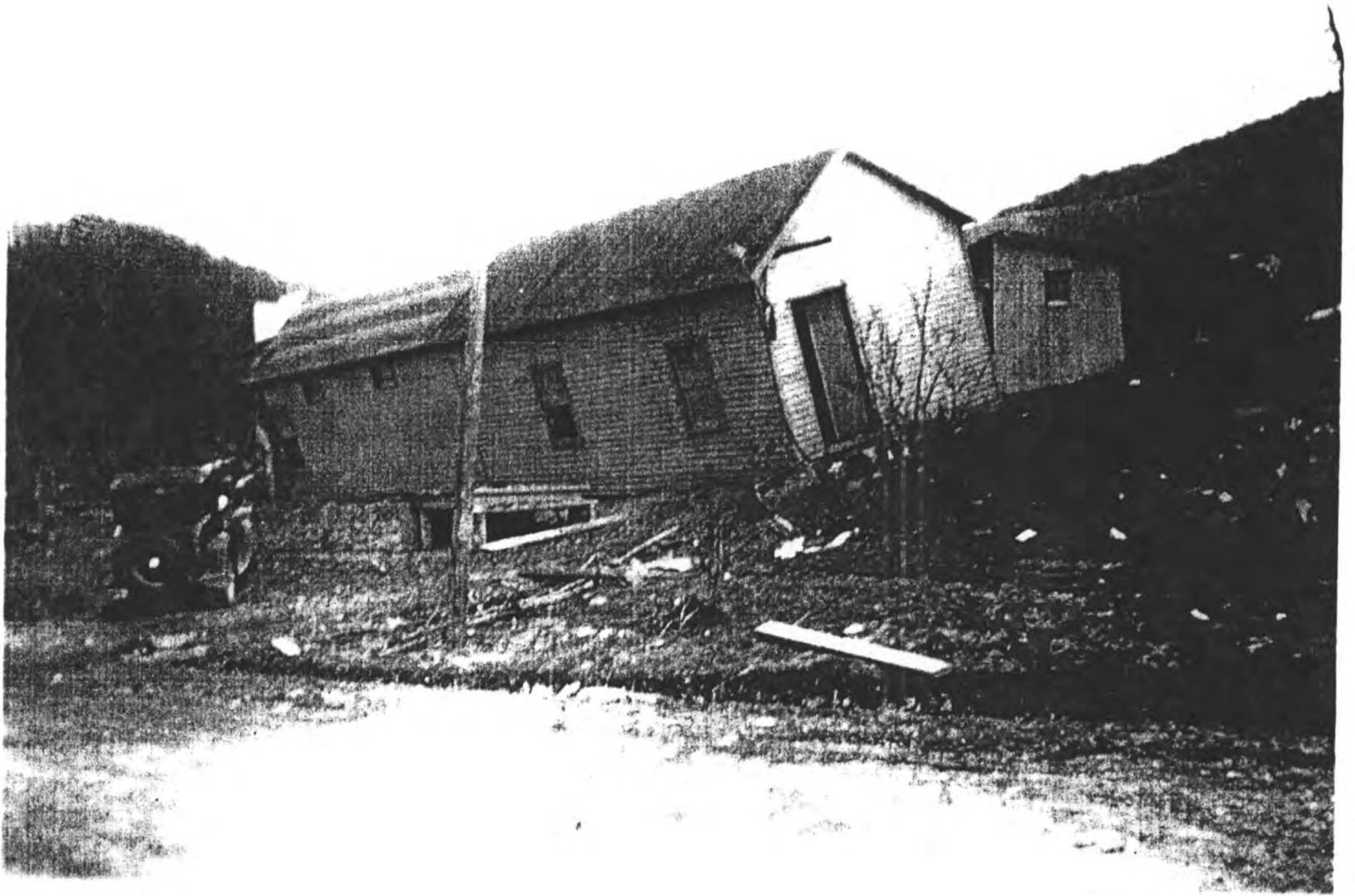
Rabbit Hash Historic District, Boone Co., KY. 1937 flood damage: floating outbuilding at rear of Rabbit Hash Ironworks.
