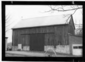
barn, north elevation
