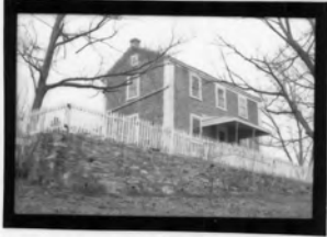
south & east elevations looking NW
