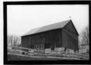
barn, south & east elevations looking NW
