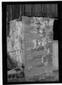
hammered stone quoins, barn foundation
