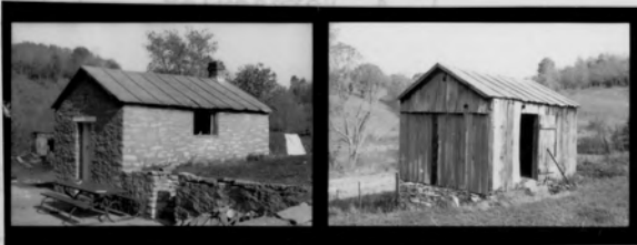
stone smokehouse and braced frame shed
