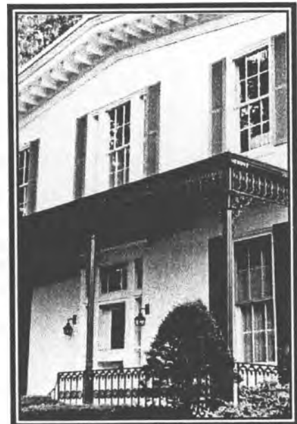
Caleb Manly built this home (KE-E-66) in the 1850s; it is now the office of the Forest Lawn Cemetery, created in the 1930s from Manly's estate.
