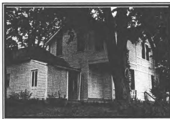
Modest as it is, this Stick Style home at 3514 Home Avenue (KE-E-98) is one of the community's most significant properties, since its exterior has been altered so little from the original.
