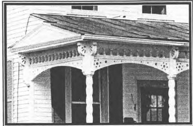
Some of Erlanger's late nineteenth-century homes, such as this handsome property at 3214 Crescent Avenue, retain their distinctive Eastlake-style porches, incorporating lathe-turned posts and balustrades.
