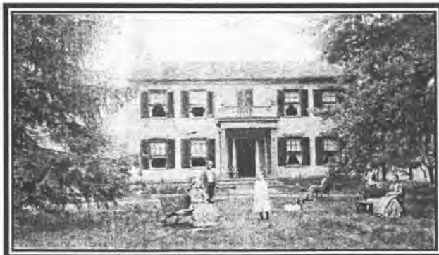
"Sugar Grove," the ca. 1826 Timberlake-Stephenson House (KE-E-71); its second story was removed following damage by a 1915 tornado.
